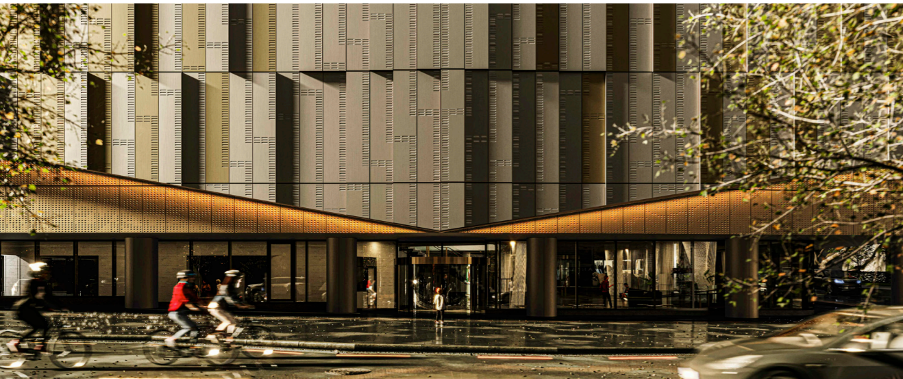
WT New Zealand Advisory Project: Heke Rua Archives Building, Wellington
